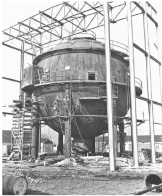
The "Eight Ball," at Camp Detrick. Airtight, bombproof, and weighing 131 tons, this one-million-liter chamber allowed Detrick's scientists to understand how aerosolized biological agents would work at different altitudes in the open air. Monkeys and human test subjects sat inside. (U.S. Army)
